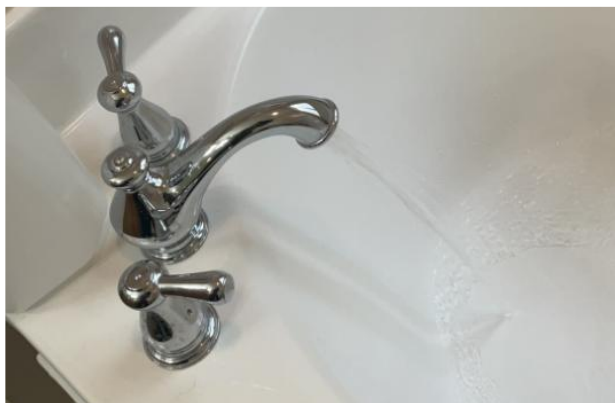
Photo 84: Functional tub faucet in master bath
