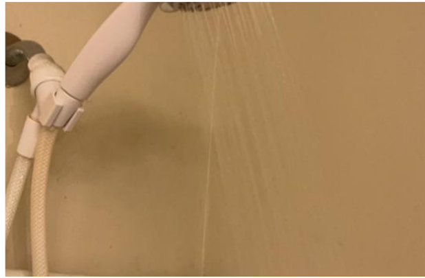
Photo 79: Functional upstairs shower
