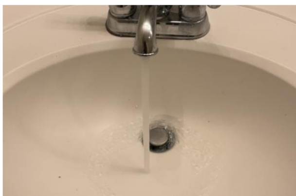
Photo 77: Functional sink upstairs bath-room
