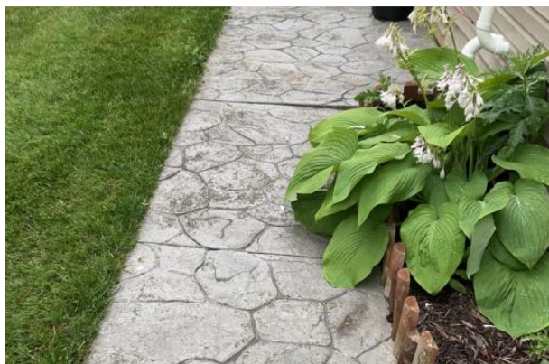
Photo 2: Side yard has a gentle slope away from the house
