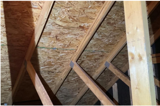
Photo 42: Attic over bedroom to the right of the stairs
