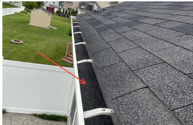
Photo 18: Granules from the shingles
