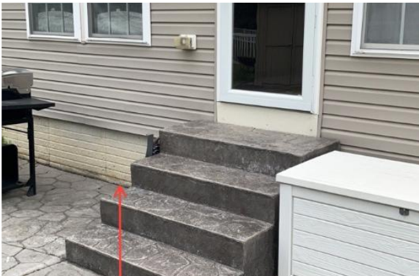
Photo 10: Missing handrail
