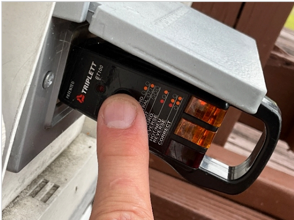
Exterior by side door
