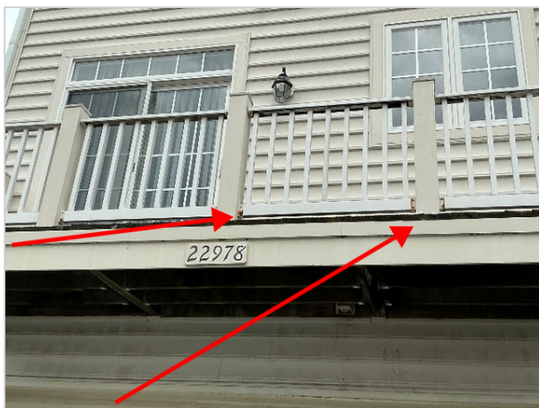
Brackets for Deck Railing
