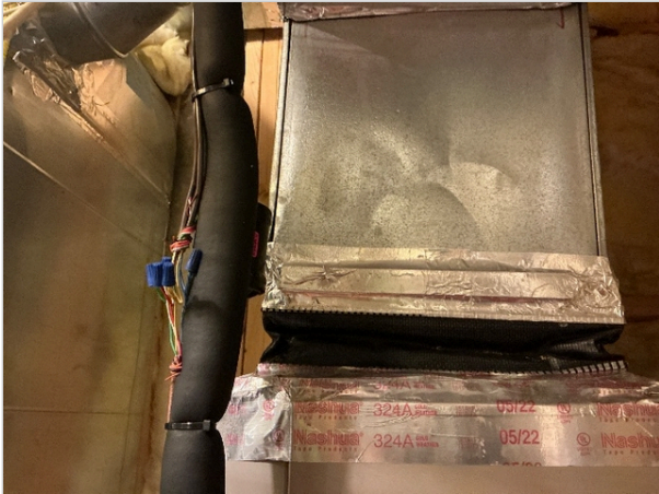
Furnace Duct Work
