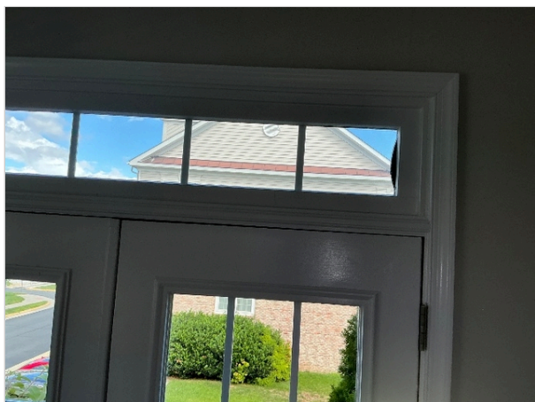
Window above living room exterior door
