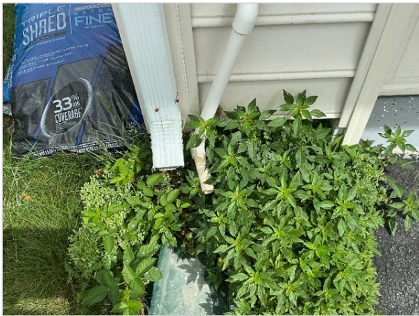
Downspout near Garage
