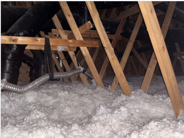
Insulation and Truss Structure
