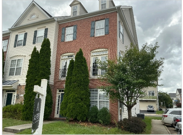
Brick Cladding on Front of Home
