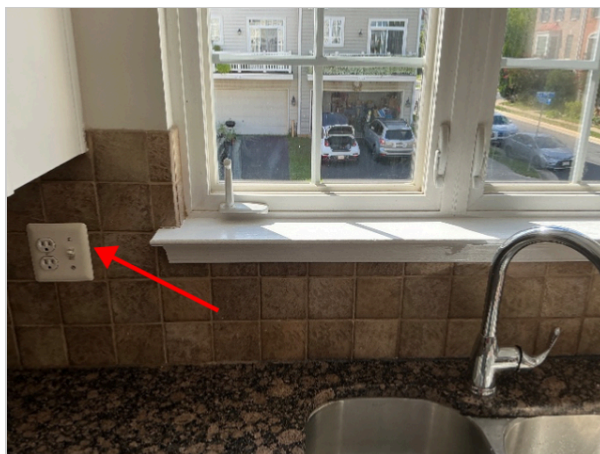
Switch to turn on disposal
