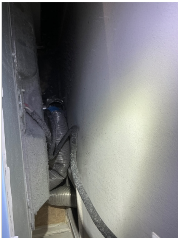
Third floor bathroom
