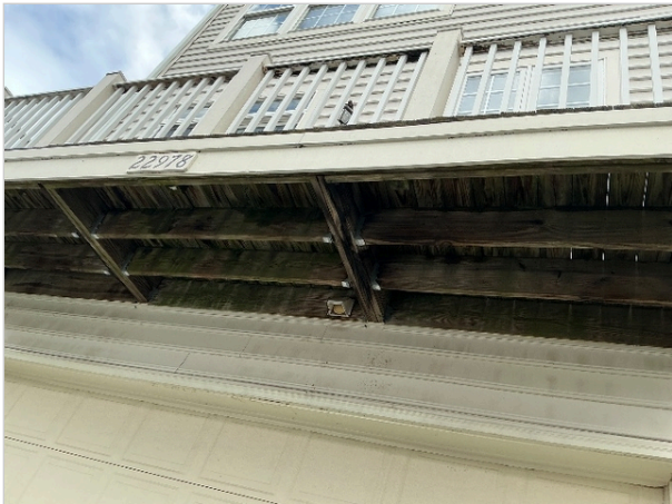
Deck / Balcony Framing
