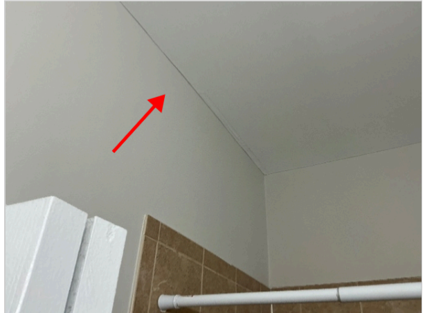
Third floor hallway bathroom
