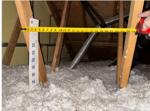
Truss Spacing
