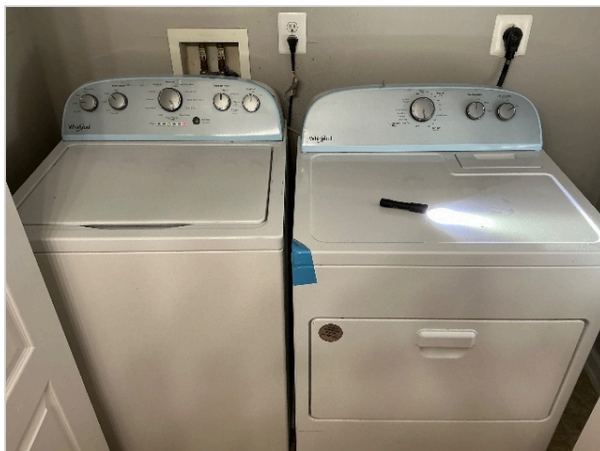
Washer and dryer located in the third floor bathroom
