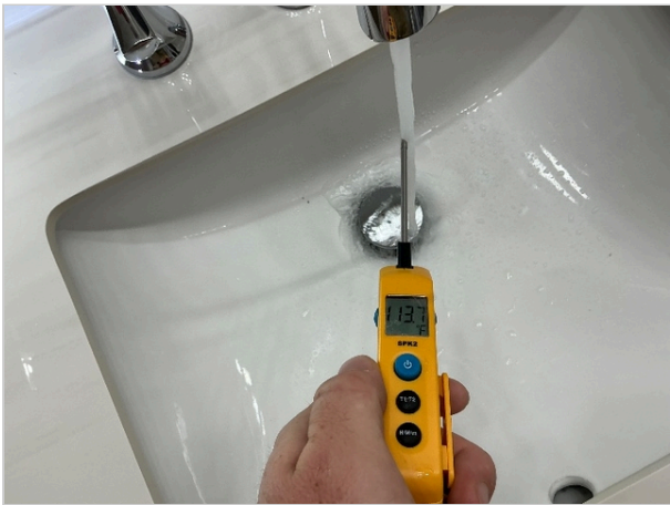
Hot Water Temp
