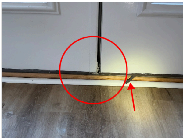
Living room exterior door
