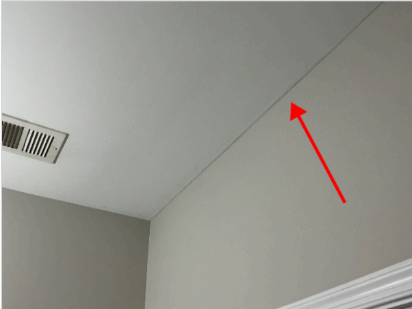
Third floor hallway, bathroom
