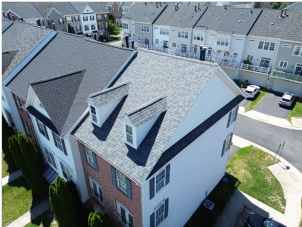
Front Side of Roof with Dormers
