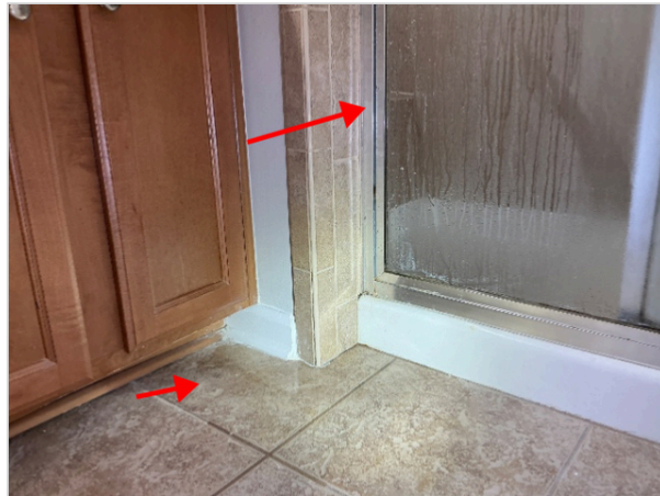
Shower in the bathroom of the third floor third bedroom
