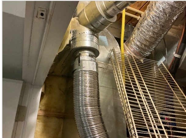
Furnace Duct Work
