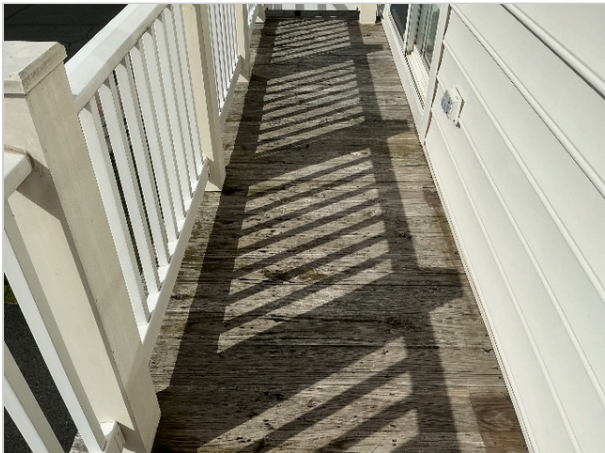
Deck / Balcony Surface
