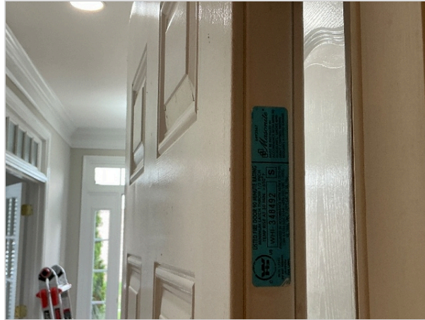
Fire rated door at garage entrance
