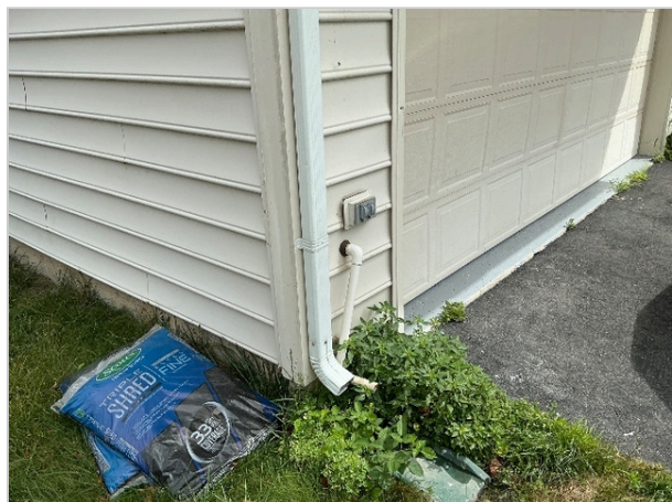
Downspout at back of home.
