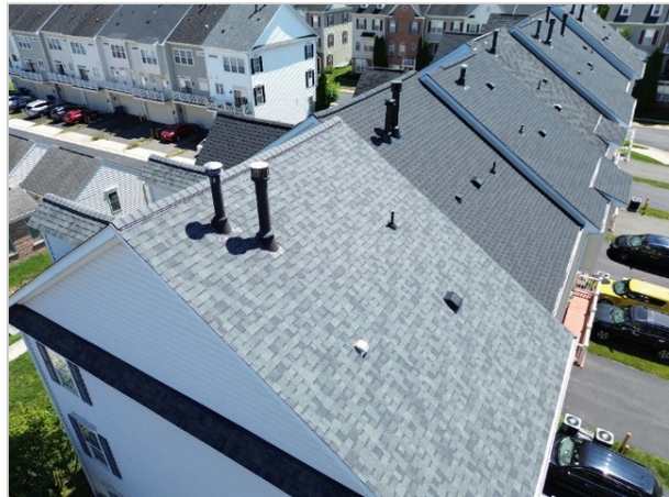
Back side of Roof with Vent Penetrations
