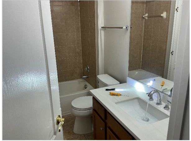
Third floor hallway bathroom
