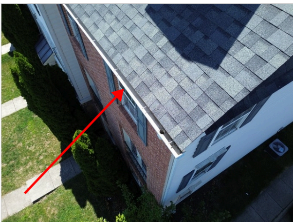
Gutters appear clear and functional
