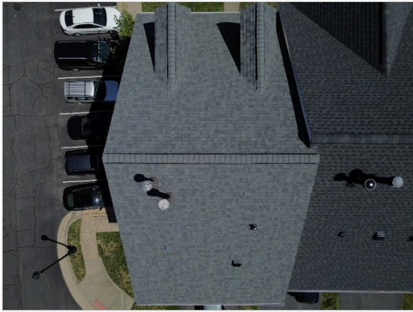
Overview of Roof
