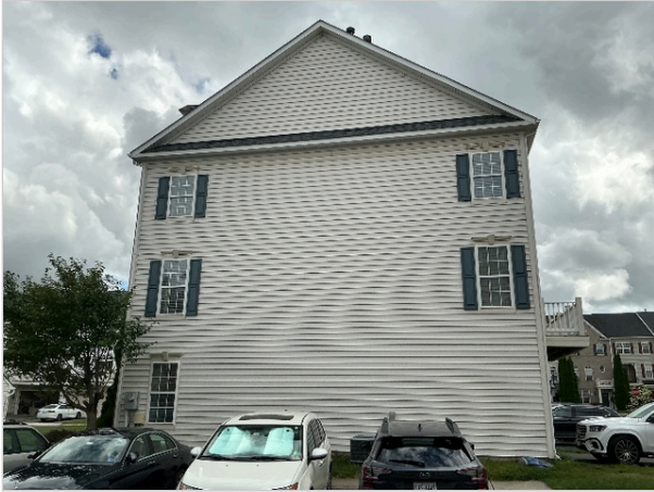
Vinyl Cladding on Side and Back of Home
