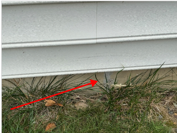
Minor repair to foundation.
