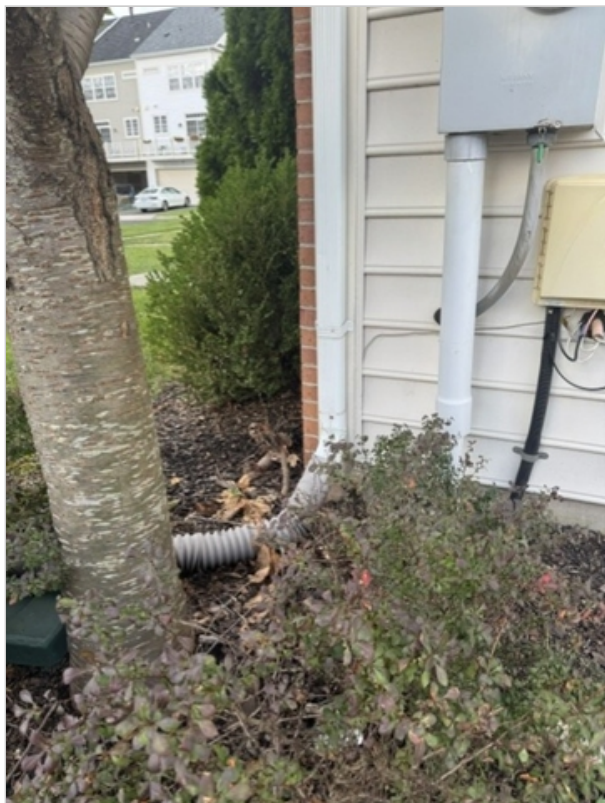
Downspout with extension
