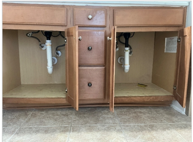
Beneath the sinks in bathroom of third bedroom
