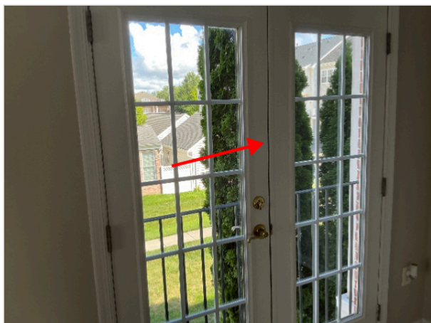
Living room exterior door
