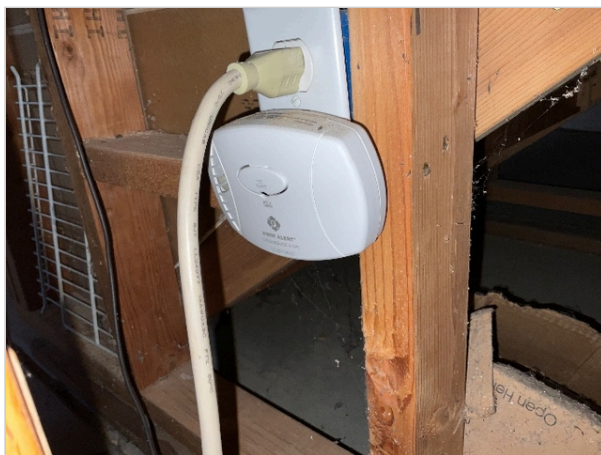
1 carbon monoxide alarm in basement only
