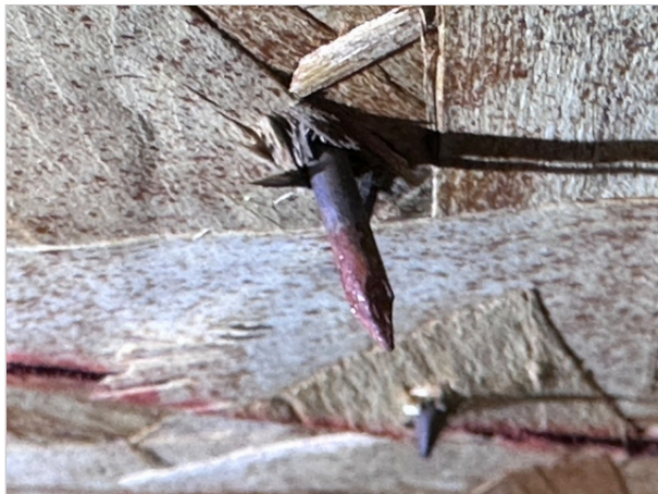
Rusted Roofing Nails
