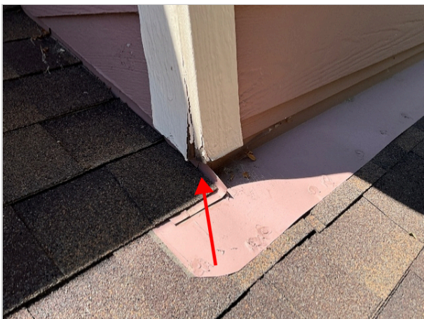
Front side of Roof
