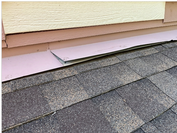
Front, right 2nd floor window
