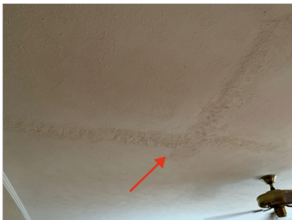
Previous repair in bedroom
