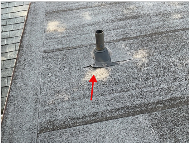
Secure plumbing boot on rear
