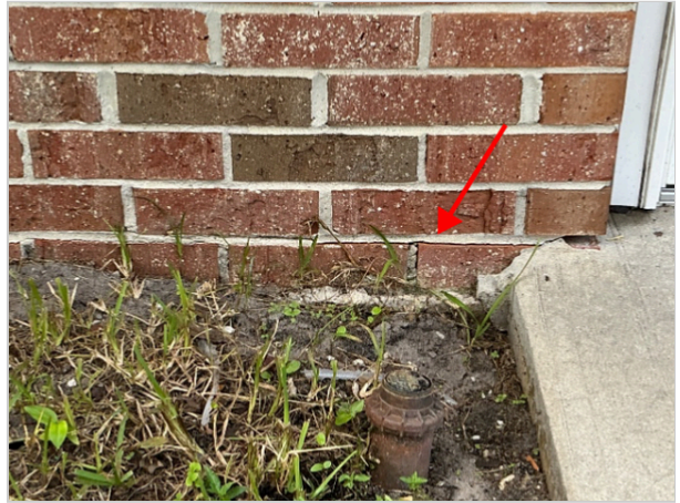
Hairline cracking
