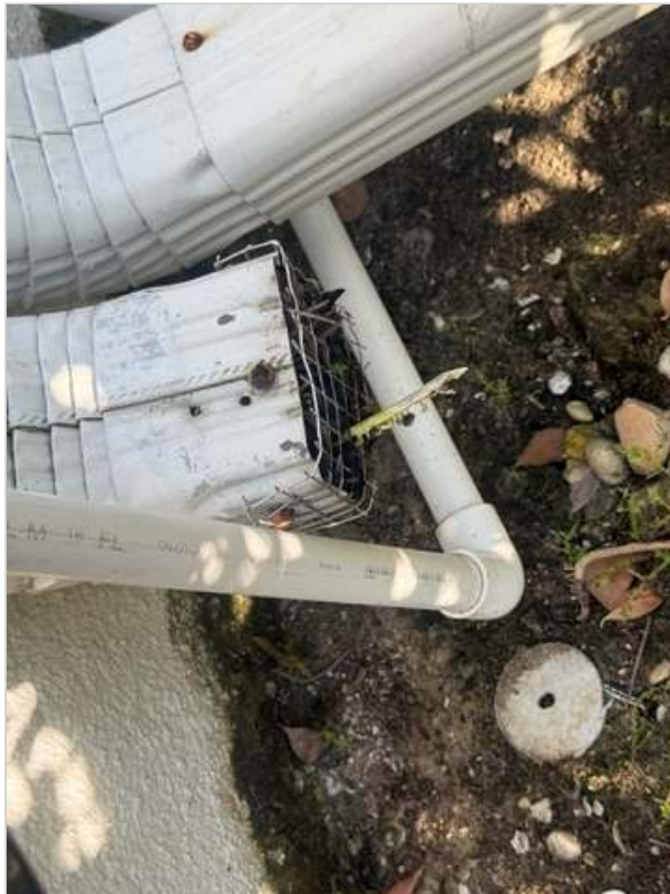
There was debris in the gutter downspout, in need of clearing.
