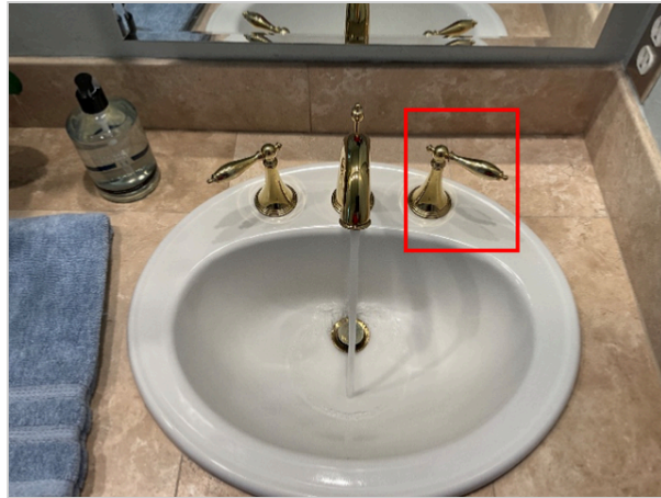
West tend hallway bathroom right side sink
