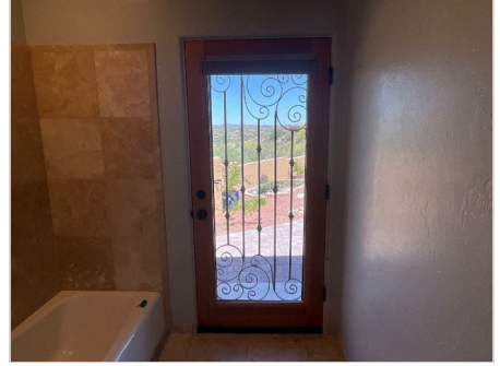
West end hallway bathroom rear patio door
