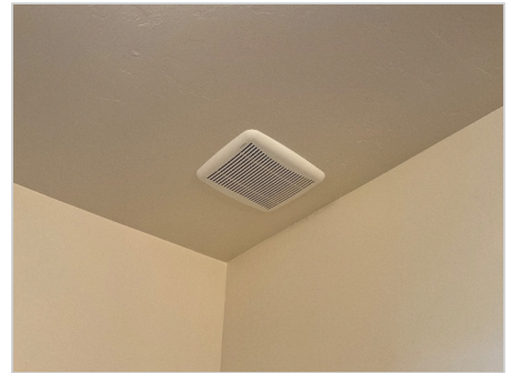
East end water closet
