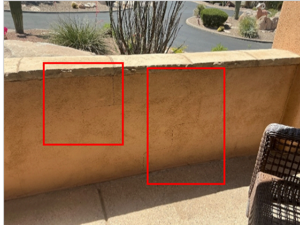
Front patio wall
