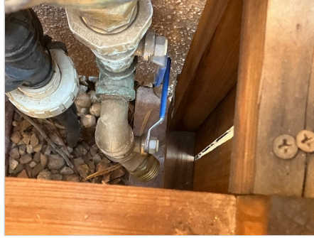
Front left of garage
