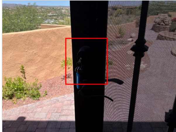
West end hallway bathroom rear patio security door
