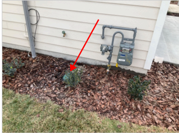
Water shut off
