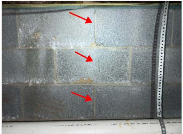
From Inside Crawlspace
