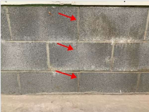
Rear Garage Wall
