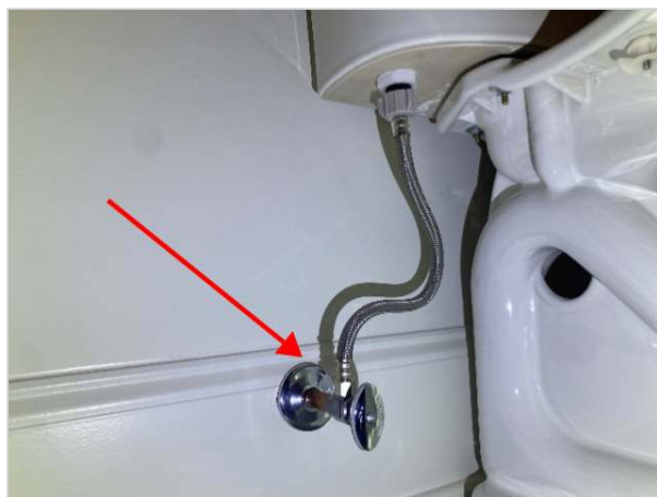
Second Floor Hallway Bathroom Toilet
