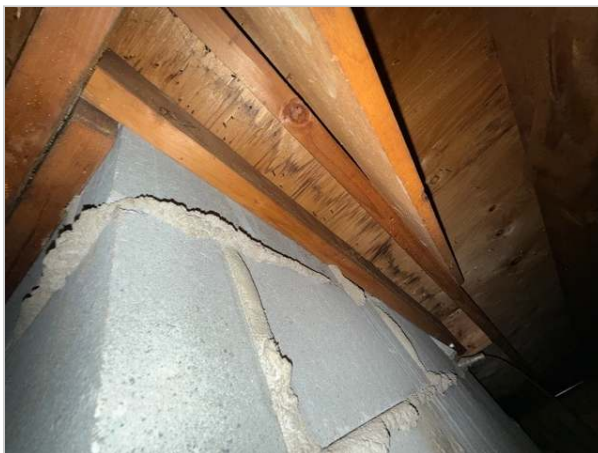
Attic above garage
