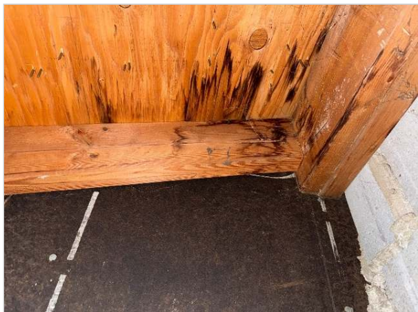
Attic above garage
