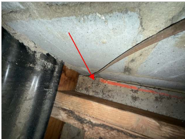
Attic above garage
