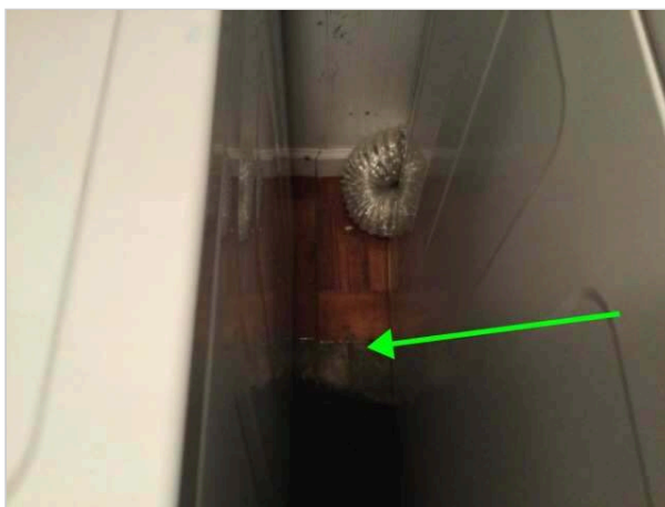
Water under the washer
