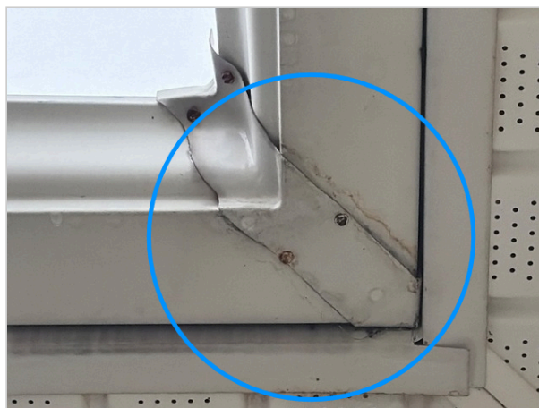
Front right side of the front door
