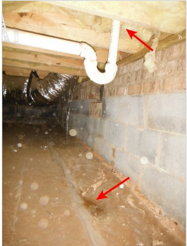
Leaking-Jetted tub
