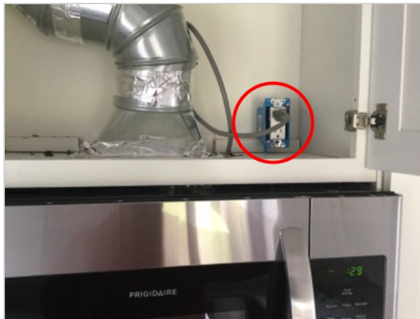
Microwave outlet above microwave
