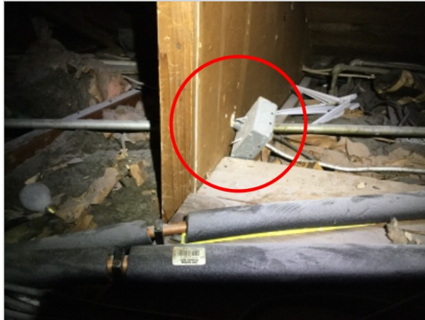
Above attic access at water heater
