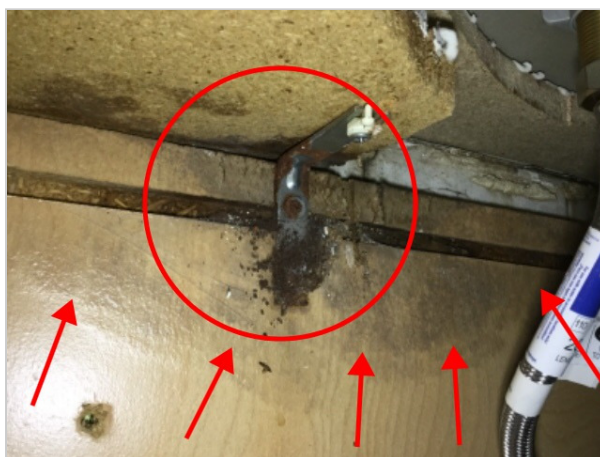
Master bathroom under sink
