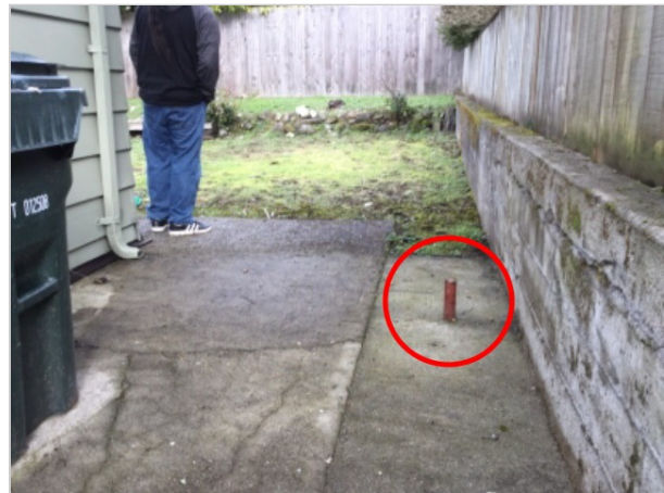
Right side yard
