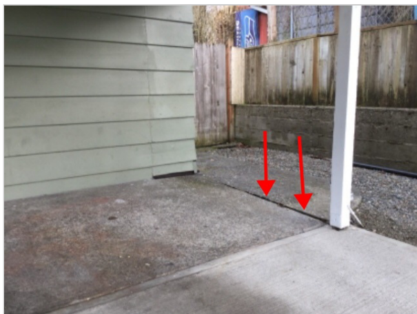
Front right walkway
