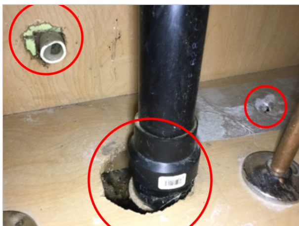
Master bathroom under sink
