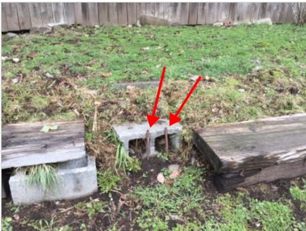
Backyard retaining wall
