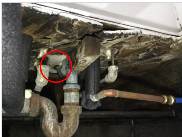
Underneath bathroom left side of house
