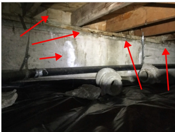
Along kitchen wall adjacent to back porch
