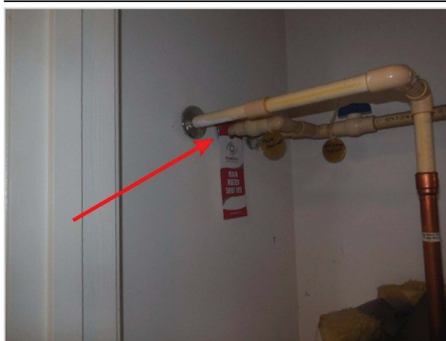
Main water shut off.
