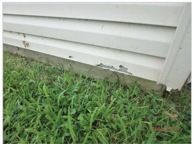
example of damaged siding
