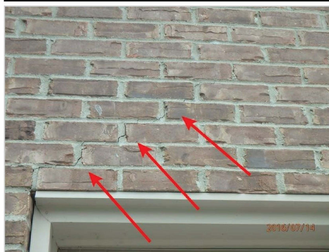
mortar crack
