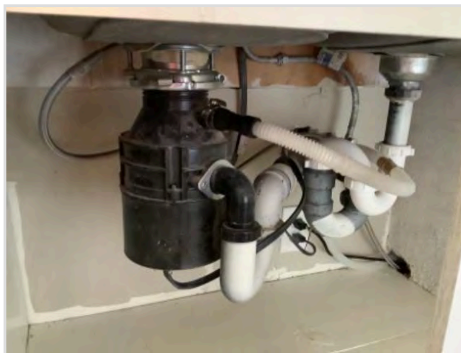
No air gap or high loop
