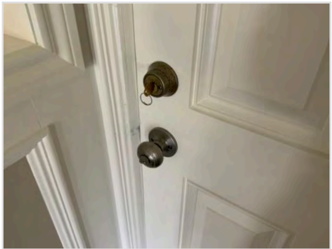
Lock keyed on the inside (back door)
