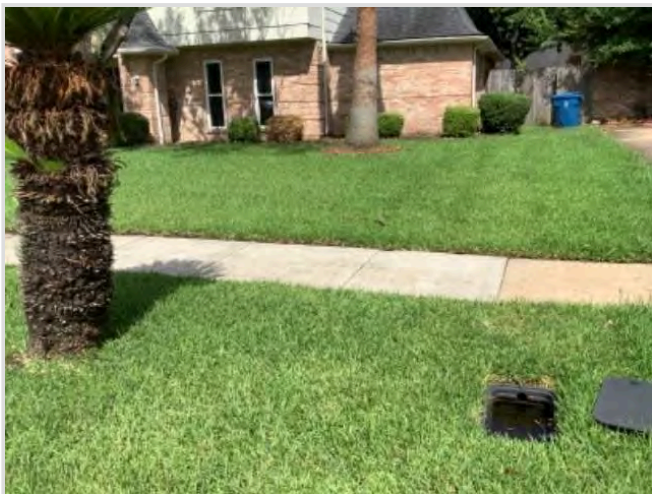
Water meter (front right side)
