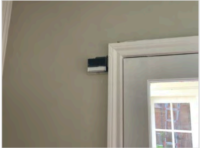
Garage door operator button (utility room)
