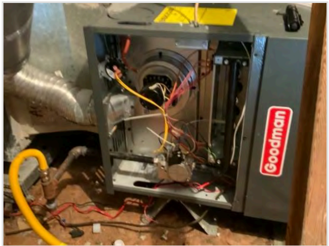
Furnace cover removed for inspection
