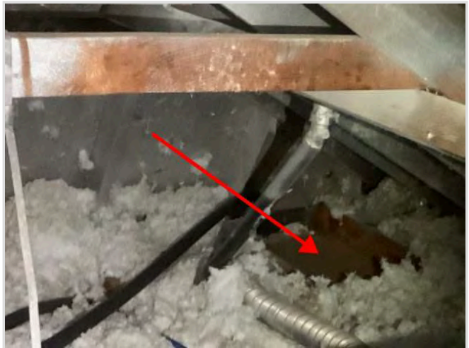
Missing insulation
