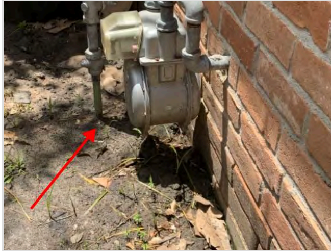
No visible bonding clamp or wire
