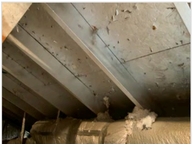
Radiant barrier was sprayed on rafters and bottom of roof decking
