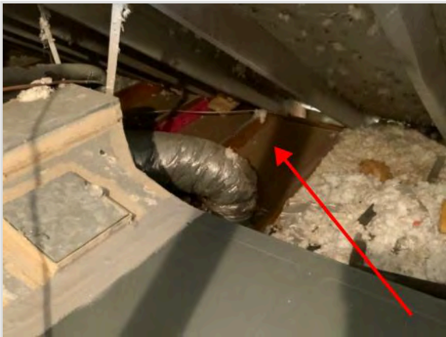
Missing insulation
