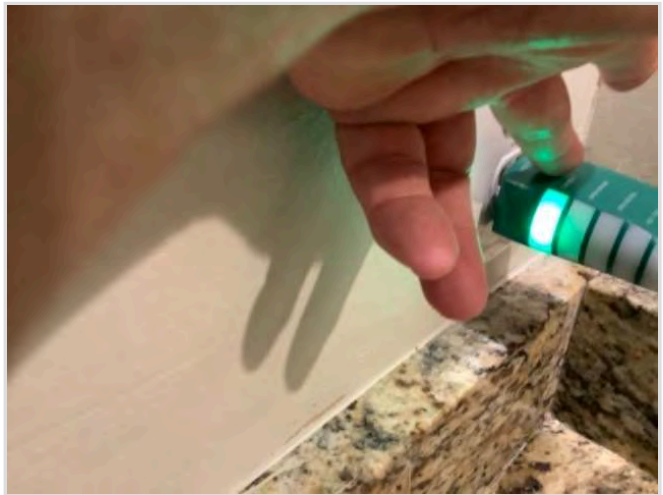
No GFCI protection (bar countertop)
