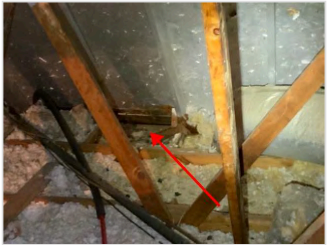
Missing insulation
