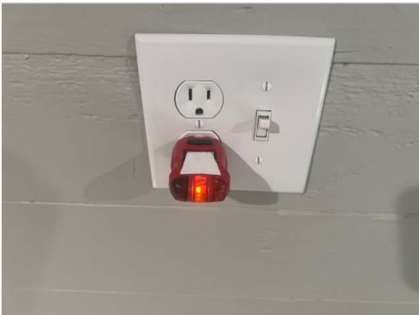
Too attic floor
