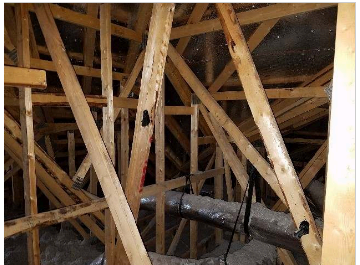
view of Texas attic space (left side).
