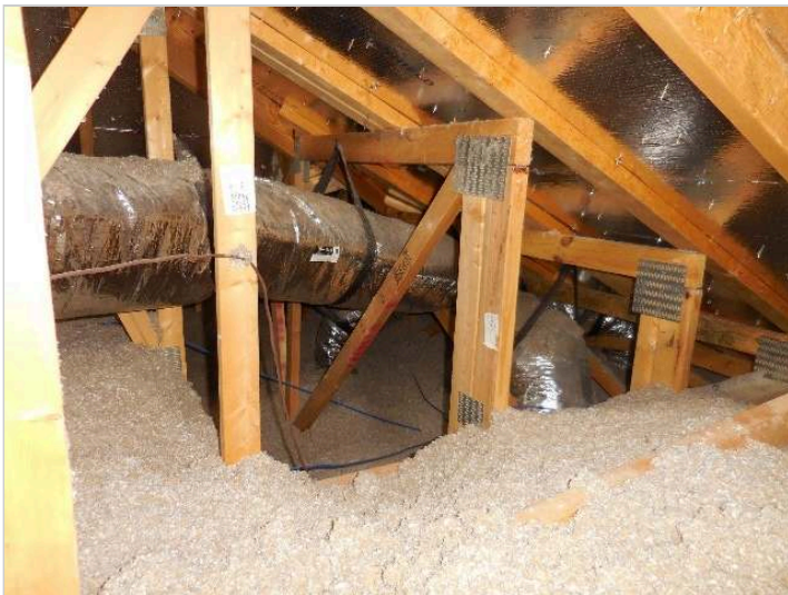
View of upper attic space (over common room).
