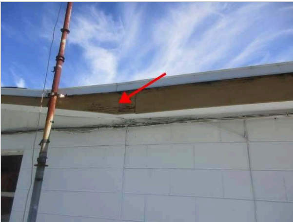
DETERIORATED FASCIA
