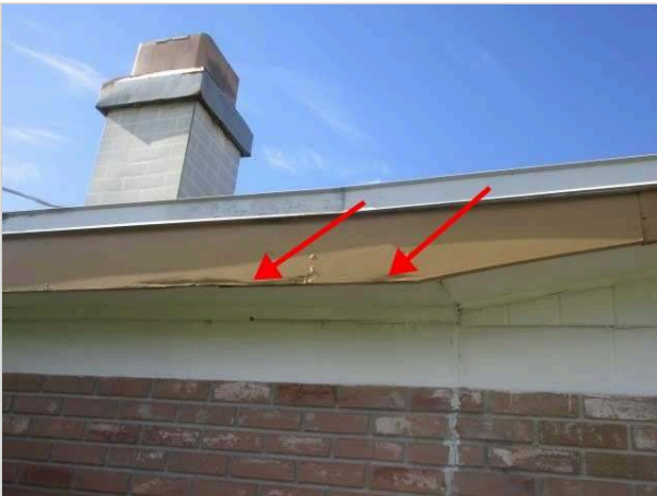
DETERIORATED FASCIA
