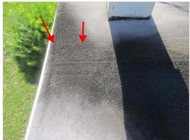
ALLIGATOR CRACKING
