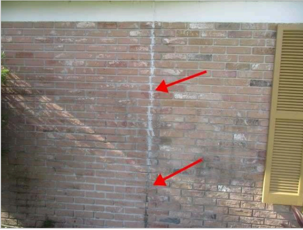
SETTLEMENT CRACK
