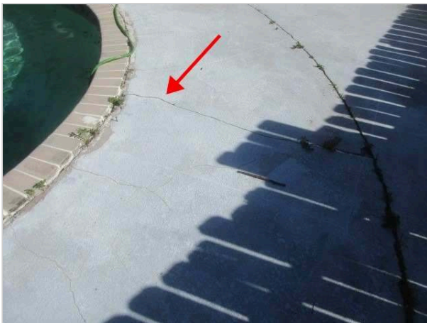
SETTLEMENT CRACKS
