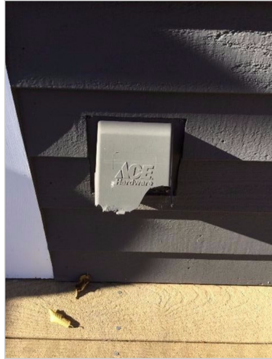
Cracked outdoor outlet cover should be replaced. Keeping moisture and water out of these outlets is important.
