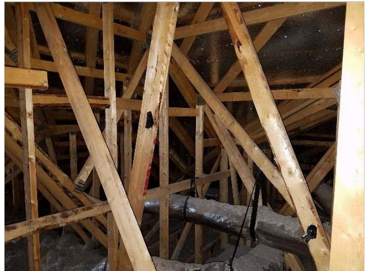
view of Texas attic space (left side).
