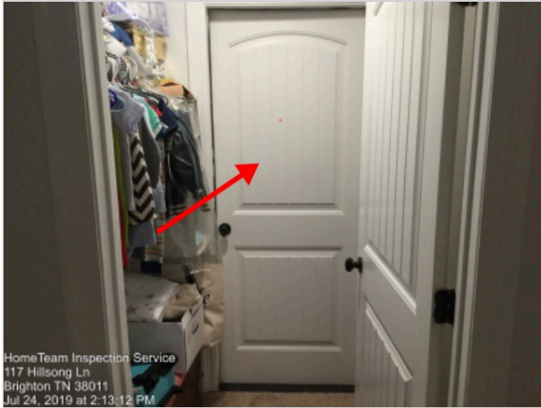
upstairs attic access
