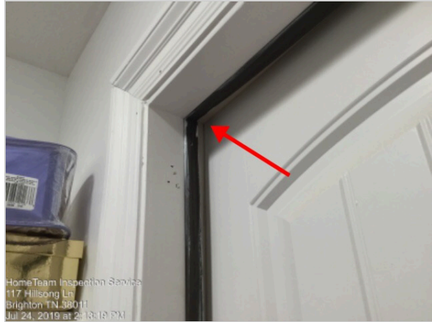
upstairs attic access
