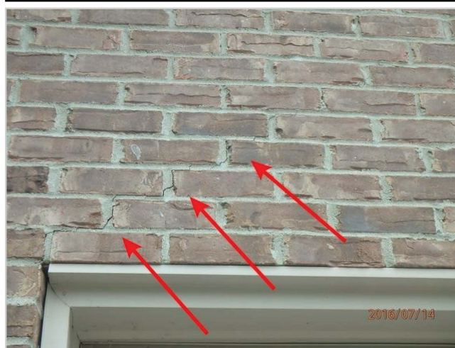
mortar crack
