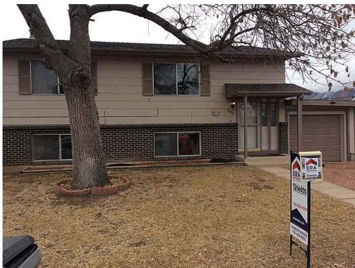
A front view of the home
