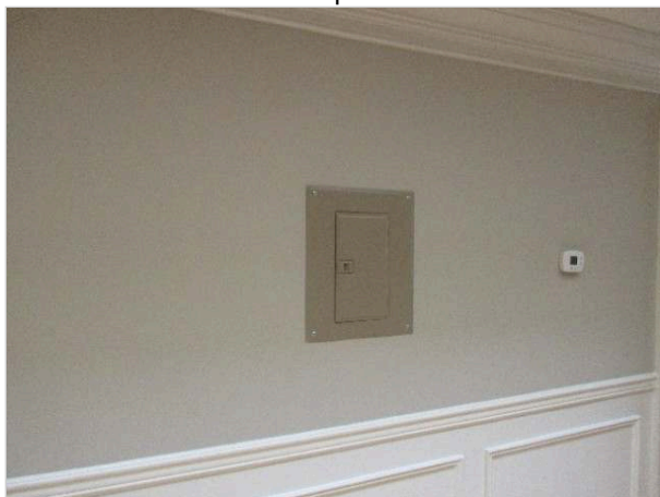
2nd floor hallway
