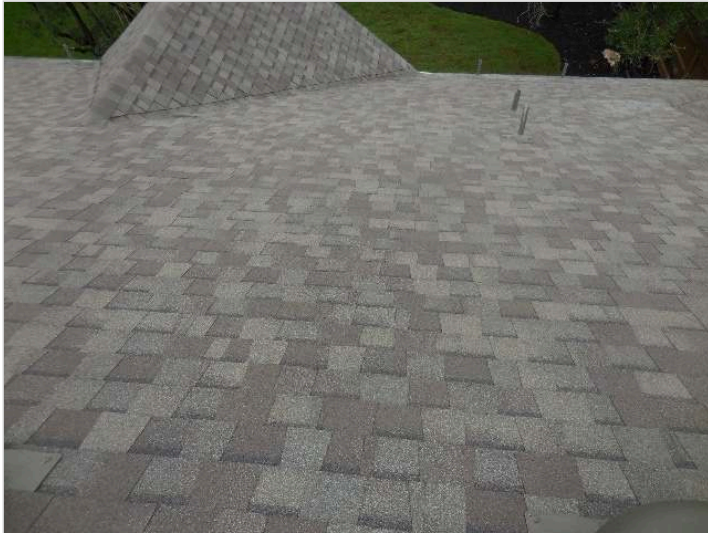
View of roof covering (back).
