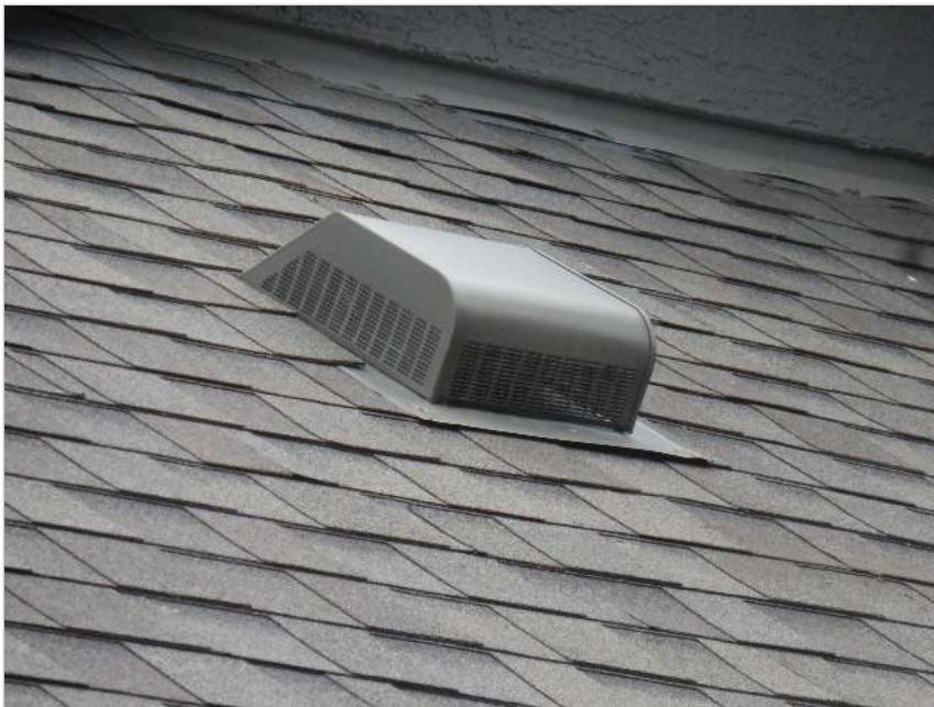
Screened dryer vent cover.
