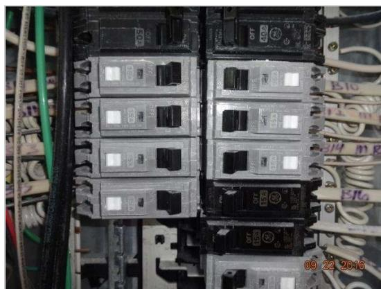
The visible wiring consisted primarily of Romex and did appear to be in serviceable condition.
