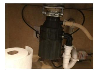
The dishwasher was tested and did appear to be functional. An anti-siphon or high drain loop was present.
