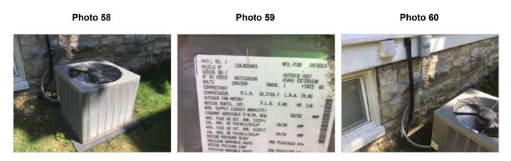
Caulk is missing from areas where cabling or tubing enters the house. Caulk helps prevent moisture from entering the home and helps keep out pests. It is recommended that the gapped areas around the areas noted below be sealed.
