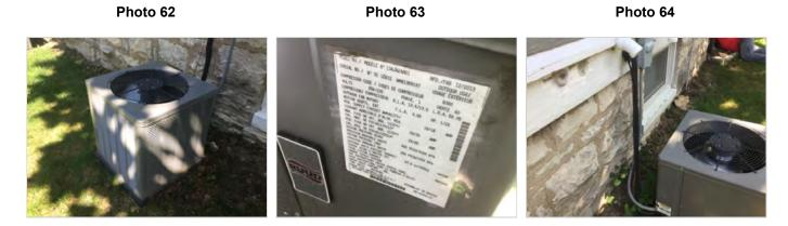
Caulk is missing from areas where cabling or tubing enters the house. Caulk helps prevent moisture from entering the
