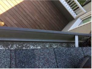
Some of the downspouts around the structure are draining into the ground with no conclusive termination point. HomeTeam recommends ensuring termination points for all downspouts is far enough from the structure and configured in such a way as to ensure water flows away from the foundation during periods of rain.
