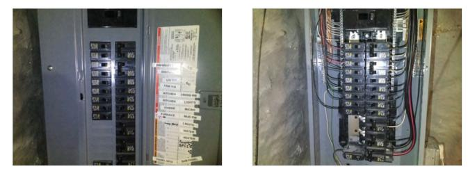
A circuit breaker in the electric panel had two attached circuits (wires). Each circuit should have its own dedicated breaker to prevent nuisance tripping and ensure good terminal contact, which may help prevent overheating. This situation is commonly referred to as a "double-tap". An electrician should repair this condition and further assess the panel for any additional required repairs.
