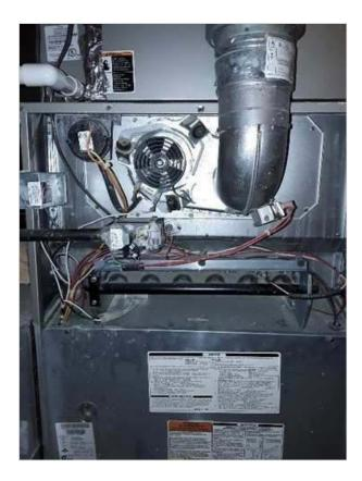
The average gas furnace will last about 15 years before needing to be replaced. A gas furnace will last longer by doing regular maintenance. The subject gas furnace has been in service for approximately 13 years and may be at or nearing the end of it's usable life.
