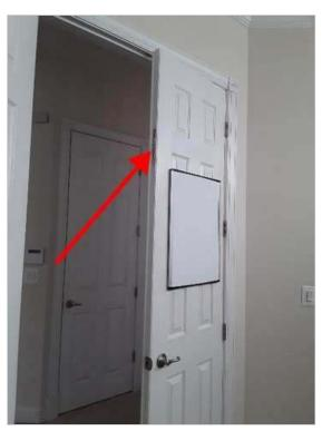
5. The french doors leading to the master bedroom did not latch properly,. This is normally easily corrected by a slight adjustment in the striker plate.
