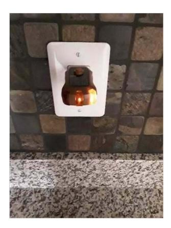
A broken switch was noted in the main level half bath. This could be a shock hazard due to exposed electrical contacts. The affected outlet(s) should be replaced by a qualified contractor.
