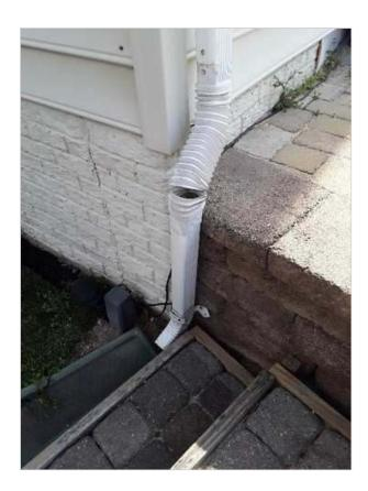
All of the downspouts were draining at or too close to the base of the foundation. All roof drainage should be directed at least six feet from the base of the foundation.
