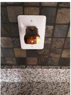
2. A broken switch was noted in the main level half bath. This could be a shock hazard due to exposed electrical contacts. The affected outlet(s) should be replaced by a qualified contractor.
