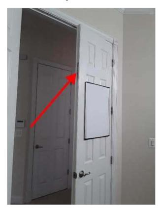
The french doors leading to the master bedroom did not latch properly,. This is normally easily corrected by a slight adjustment in the striker plate.
