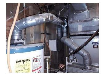
Most tank-type water heaters last 10 to 20 years, with the average age of replacement between 12 and 14 years. The age of the water heater was approximately 14 years old and was most likely at or nearing the end of its useful life.
