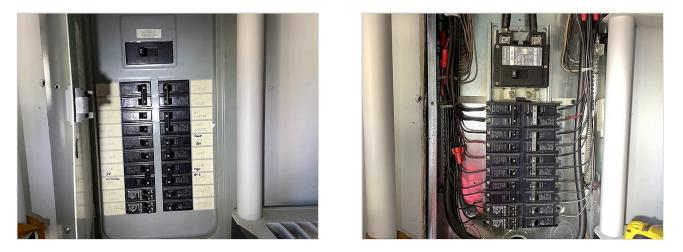
The visible house wiring consisted primarily of the Romex type and appeared to be in good condition. An electric service grounding system was installed. Service grounding requirements have changed many times over the years. The grounding system for a 30-year-old electric service is different from that of a 10-year-old service. The inspection does not attempt to verify that the grounding system or any other part of the electric service complies with current codes.
