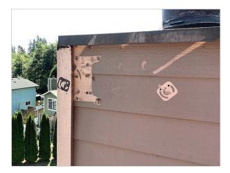
The metal flue chase cap is rusted. Over time, this may lead to water intrusion. No points of visible water intrusion were evident, although our view was limited. As a maintenance item, the rust should be removed and the metal cap painted and sealed to help prolong the life of the cap and reduce the potential for water intrusion.
