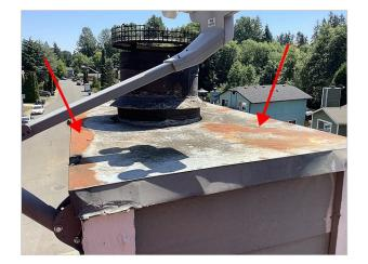
**The chimney is missing a rain cap**. A rain cap should be installed to prevent excessive water intrusion and deterioration of the chimney and its components.
