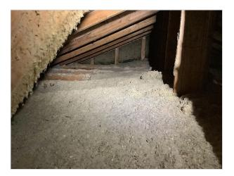
**Parts of the attic show signs of previous water intrusion.** The areas were dry at the time of the inspection. Multiple moisture readings were taken and reading were lol below 6% moisture content. The buyer should maintain vigilance in monitoring the areas for any recurrence of the previous issue and should rectify any issues immediately upon observing them.
