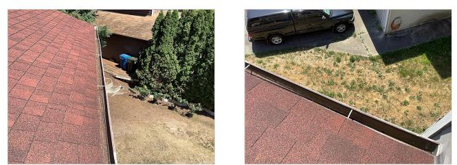
**Gutters were in need of repair** at the time of the inspection. Clogged or damaged gutters can cause roof drainage water to drain at the base of the foundation, causing basement water problems. Overflow from gutters can cause damage to fascia that is not visible or apparent at the time of the inspection. The gutters should be repaired.
